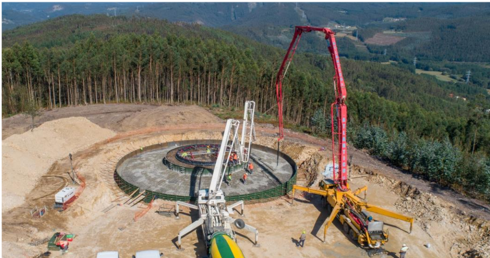
(1) Construction of Miñón wind farm (A Coruña). Materials collection (2) Construction of Oural wind farm (Lugo). Foundations
